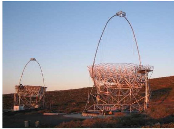
Figure 2: In the foreground the second MAGIC telescope. The structure is already fully installed. In the background the first MAGIC telescope which has been in scientific operation since summer 2004.
