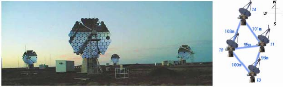
Figure 1. The CANGAROO-III telescope system near Woomera, South Australia viewed from the south. The drawing on the right shows the arrangement of the four telescopes.
