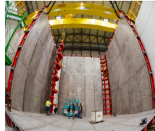
November 2016, cryostat structure assembly
