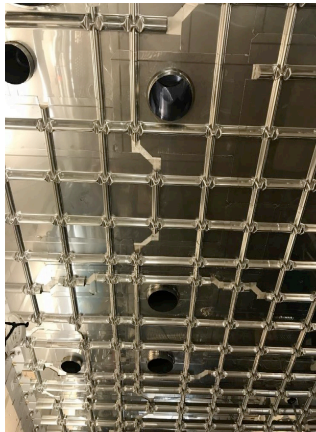
Custom pieces on roof, around penetrations
