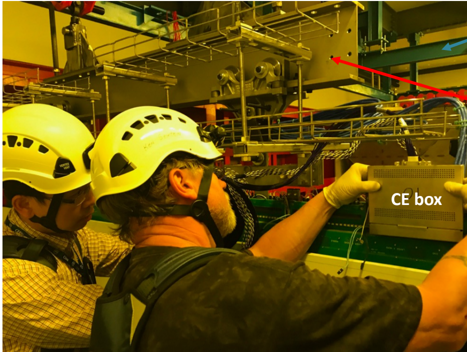
Installation of Cold Electronics (CE) boxes on top of APA frame
